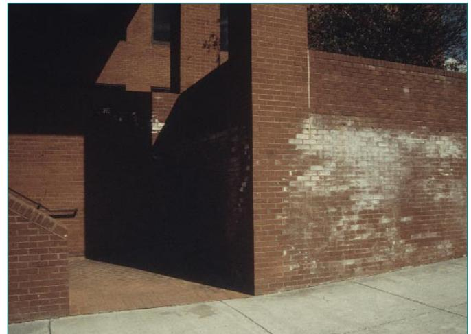
*Figure 1. Efflorescence is often called "new building bloom" because it appears on fresh masonry surfaces. (IMG14593)*
