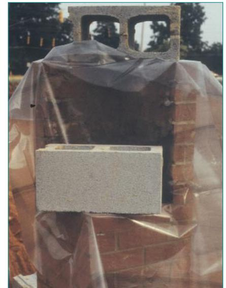
**Figure 4.** The top of masonry walls should be protected with a tarp whenever rain or snow is expected. It is good practice to cover work at the end of each day to help keep excessive water out and aid curing. (IMG15557)
