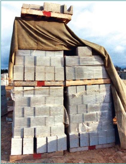
**Figure 3.** By placing masonry units on pallets and covering them with tarps, it is possible to keep them dry while stored at the job site. (IMG12505)
